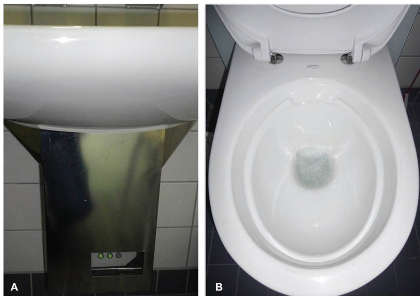
Figure 2. Hygiene siphon and rimless toilet. The Hygiene siphon uses vibration (50–200 Hz), high temperatures (85°C), and ultraviolet light to prevent biofilm formation. It is covered to discourage a frequent change of settings and for cleaning and disinfection purposes.
